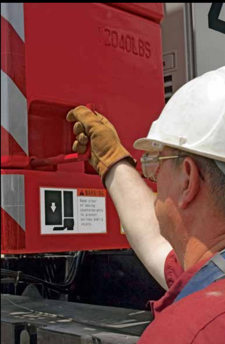
Pull counterweight pin & lower counterweights to ground
